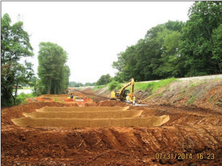
P-5206 Reid to N. Kannapolis - Erosion Control
