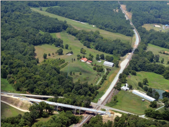
C-4901 Bowers to Lake - Turner Road Bridge
