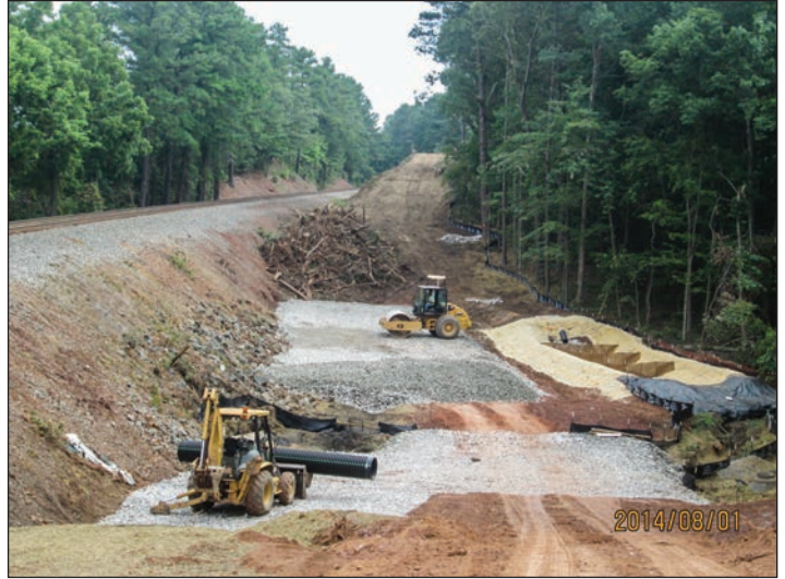
P-5201 Morrisville Parkway, west approach to bridge
