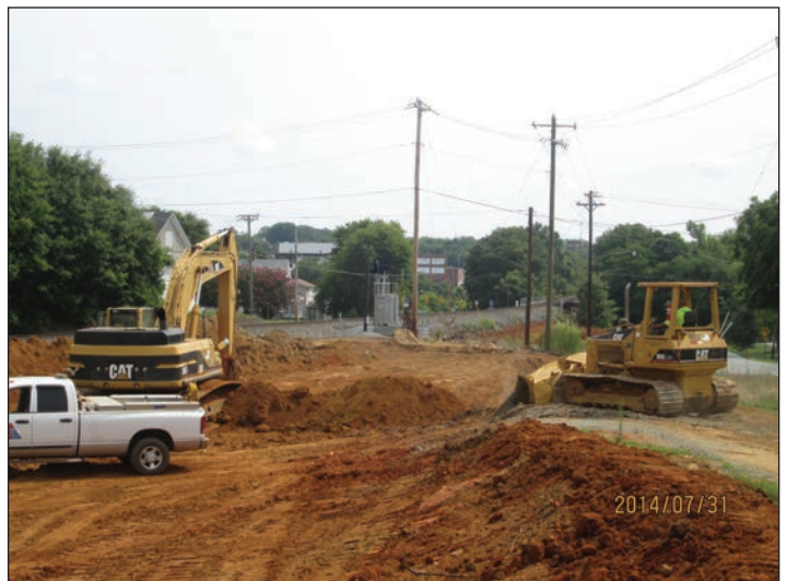
P-5205 Graham to Haw River Grading
