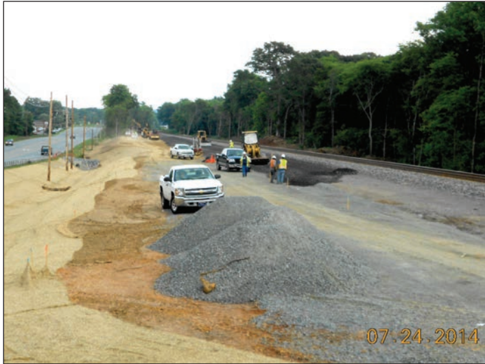
P-5208 Haydock to Junker - grading
