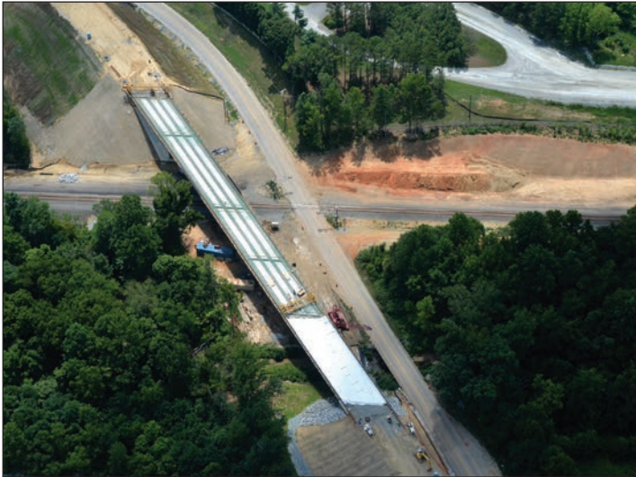
C-4901 Bowers to Lake - Upper Lake Road Bridge
