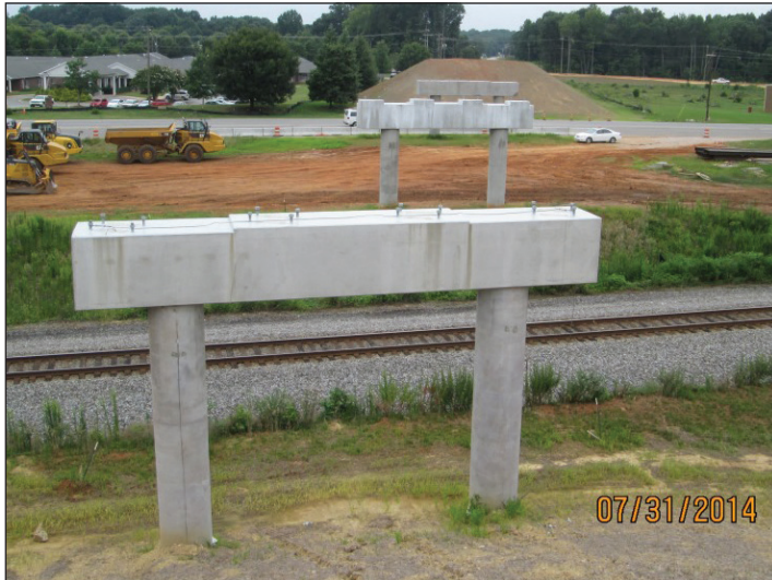
P-5206 Peeler Road Bridge Construction
